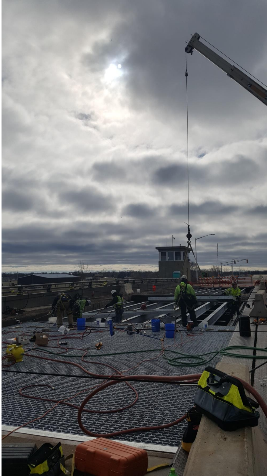
Figure 1: Independence Bridge Construction (Looking South)
