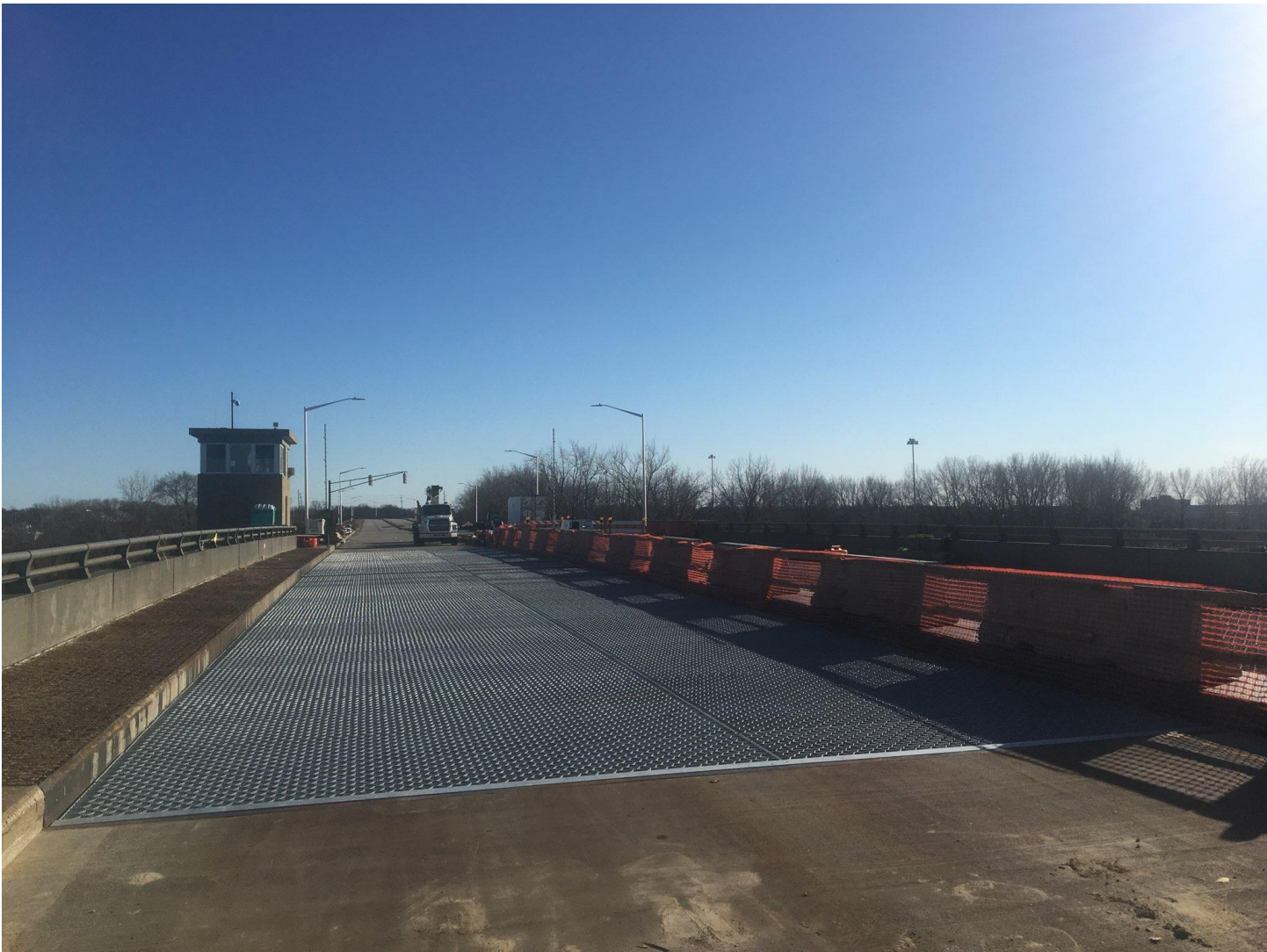
Figure 2: Independence Bridge Construction Northbound Complete (Looking South)
